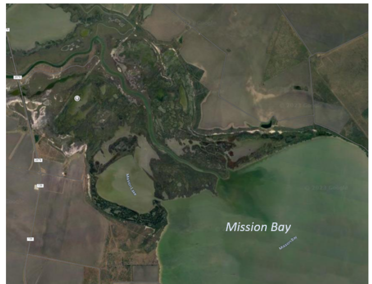
Mission River Living Shoreline Restoration
